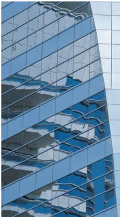
Due to its selective cooling process, AAG-dur has a less distorted surface flatness and a better optical quality than AAG-safe, making it the preferred choice for the heat-treatment of highly reflective glass-types and further processing such as lamination.
