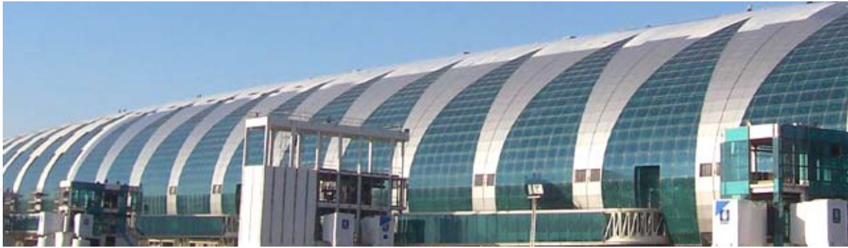
Dubai International Airport Concourse 2 with AAG-screen
